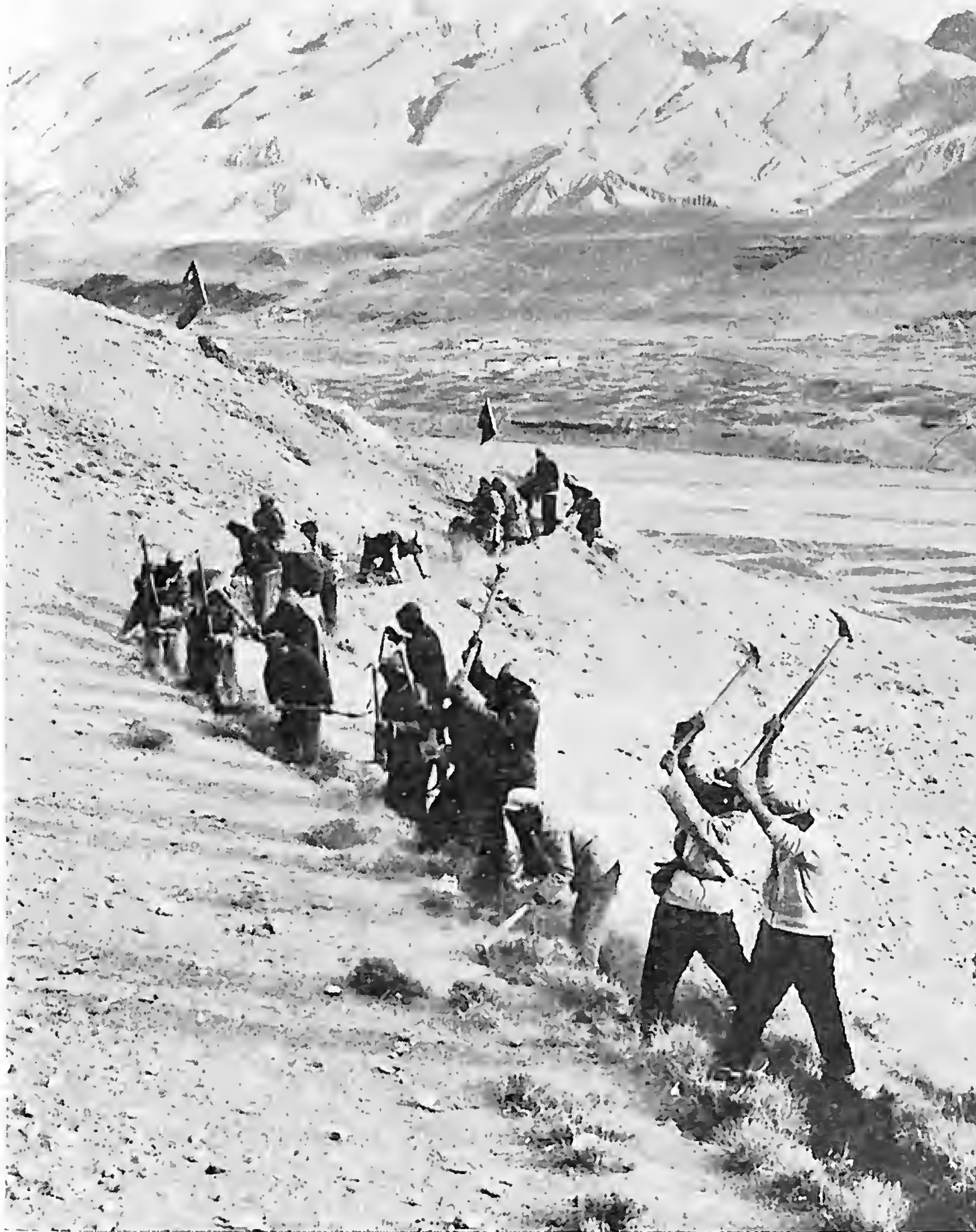
Digging ditches on the slopes.
